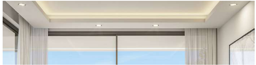
LED spot light & cove lighting
